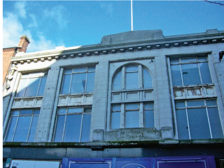
Above / Derelict Art Deco building on North Street
